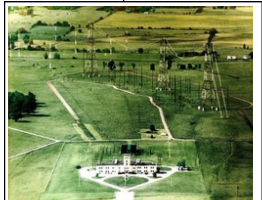
Siege guns: VOA-Bethany's six transmitters were connected to dozens of large antennas spread across a 1-square-mile area. Many people may recall seeing these towers as they drove past on Interstate 75.
