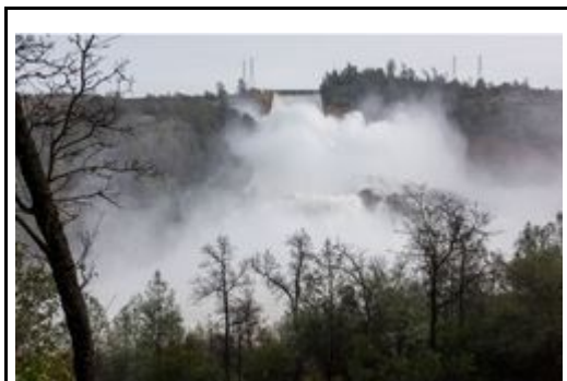
The California Department of Water Resources released 100,000 cubic feet per second from the damaged spillway to decrease the lake level by 50 feet to handle the next round of storms expected this week.
