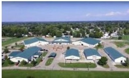
An aerial view of the Greene County Fairgrounds and Expo Center, the new home of Hamvention. [Greg Ordy, W8WWV, image]
