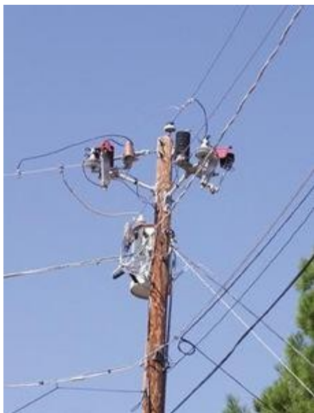
The "old" BPL technology, seen here, employed frequencies in the HF range.
