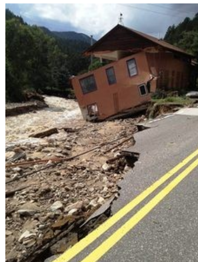
Road and property damage in Jamestown, Colorado [Boulder County photo]
