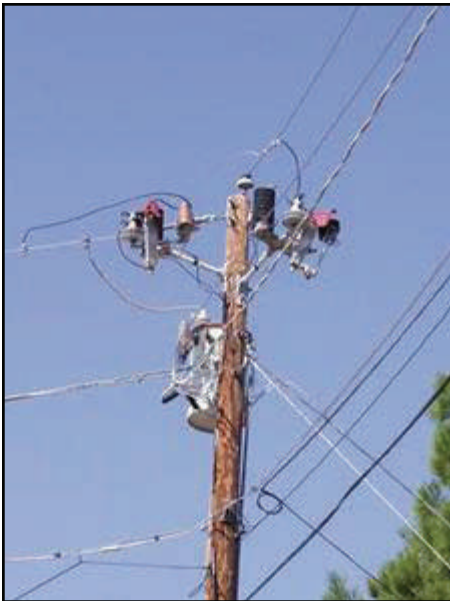
BPL technology uses the electricity grid in a city and the wiring in individual homes to provide direct "plug in" broadband access through electricity sockets, rather than over phone or cable TV lines.
