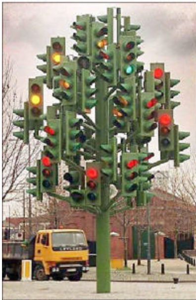
New traffic signals installed in downtown Salt Lake City, to help with the traffic congestion during the Winter Olympics....
